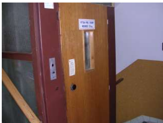
Nerudova 20, 22 – prosklená šachta
